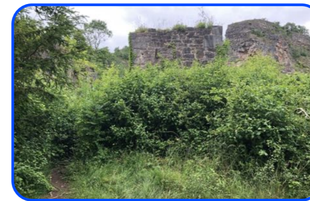
Welsh Brake House Front View
