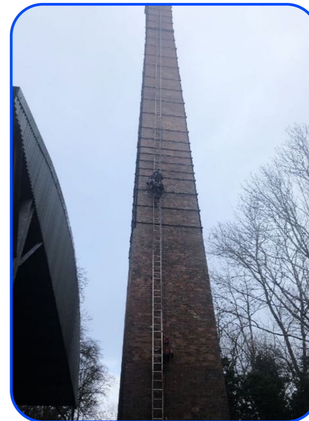
Steeple Jacks at work on the Hoffmann Kiln
