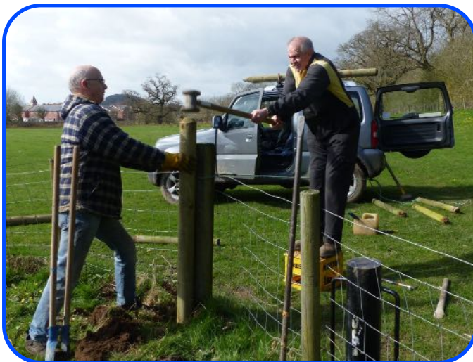
Maintaining the Fences
